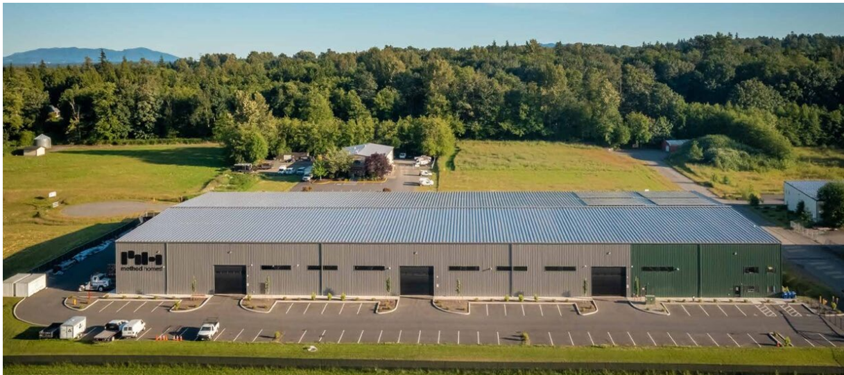
Figure 21. Method Homes – Ferndale, WA, Built 2021
