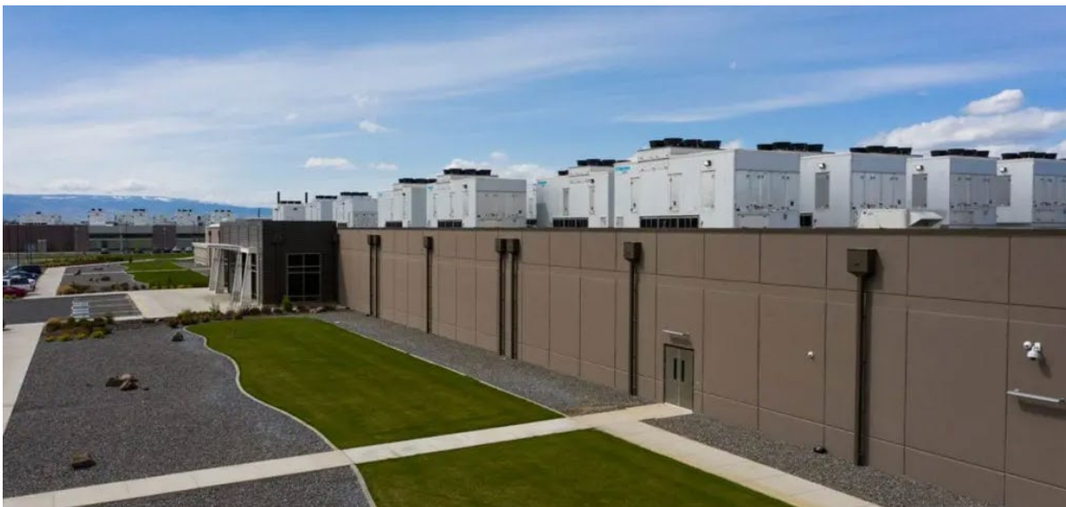
Figure 11. Sabey Data Center - Quincy, WA, built in 2022
