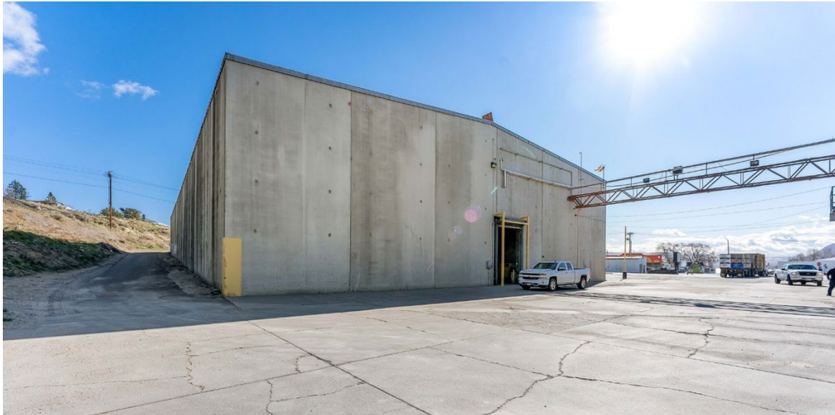
Figure 20. Gebbers Farms Cold Storage, Quincy, WA
