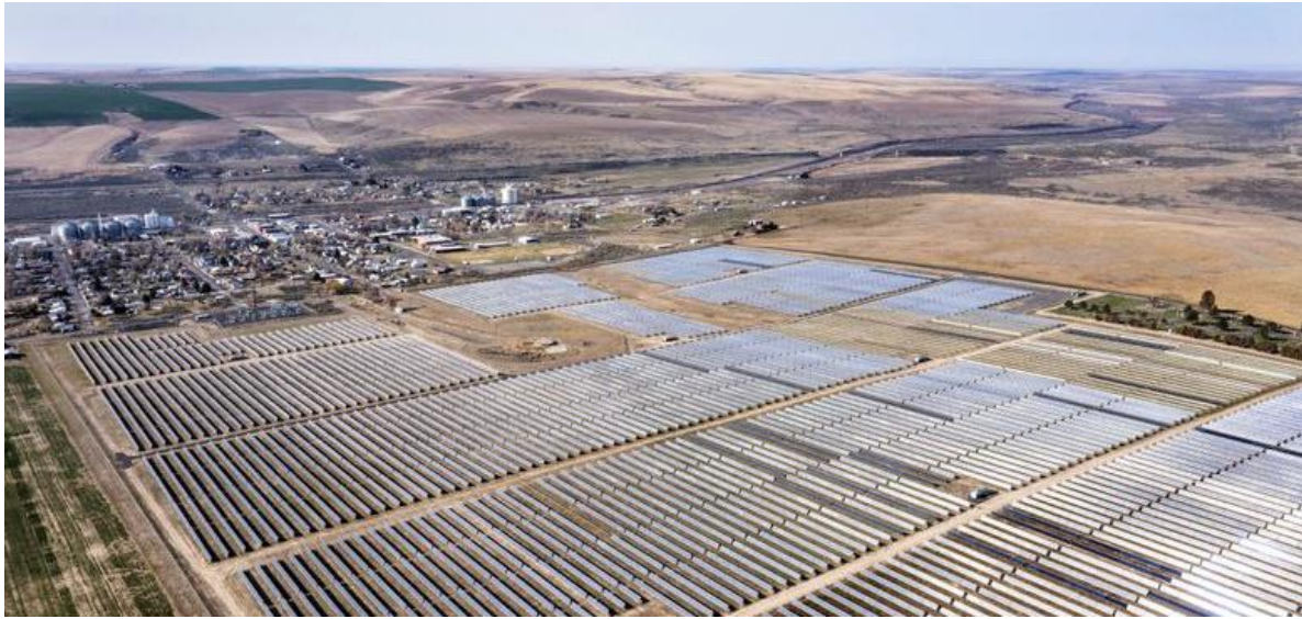
Adams Nielson Solar Farm, Lind, WA (28 mW / 200 ac / 4,000 homes)
